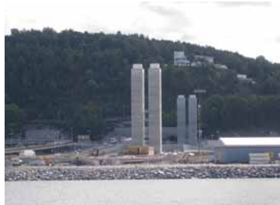
The Bjørvika tunnel during its construction
