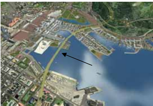
Illustration of the Bjørvika tunnel, the subsea tunnel in the Oslo harbor
